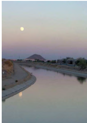
This Central Arizona Project aqueduct carries water from the Colorado River to Tucson
